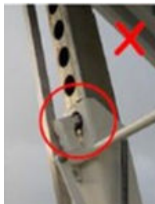
Figure 4-27: Pawl lock is NOT engaged correctly.
