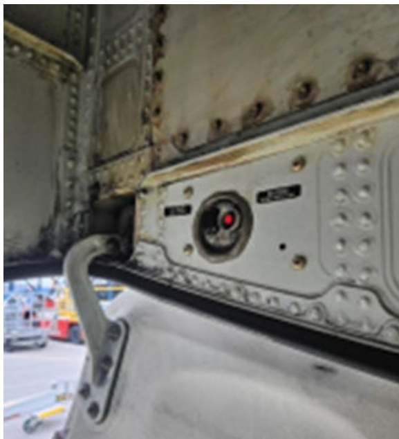
Right hand side service panel. NOTE; this is 2.5m above ground level.
