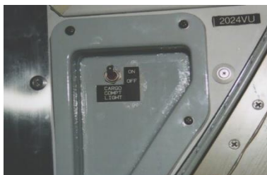
Light switch beside the hold door (Aft hold)
